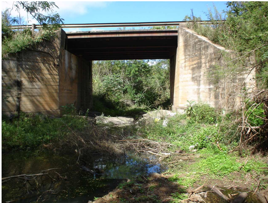
View of the current bridge structure, abutments and decking
